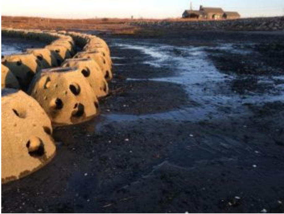
This photograph was taken in January 2017. The artificial reef is functioning as designed; fine grained sediment is being deposited across the project area, which is necessary for the establishment of marsh vegetation. As the next phase of the project, marsh vegetation will be planted in spring 2017.
