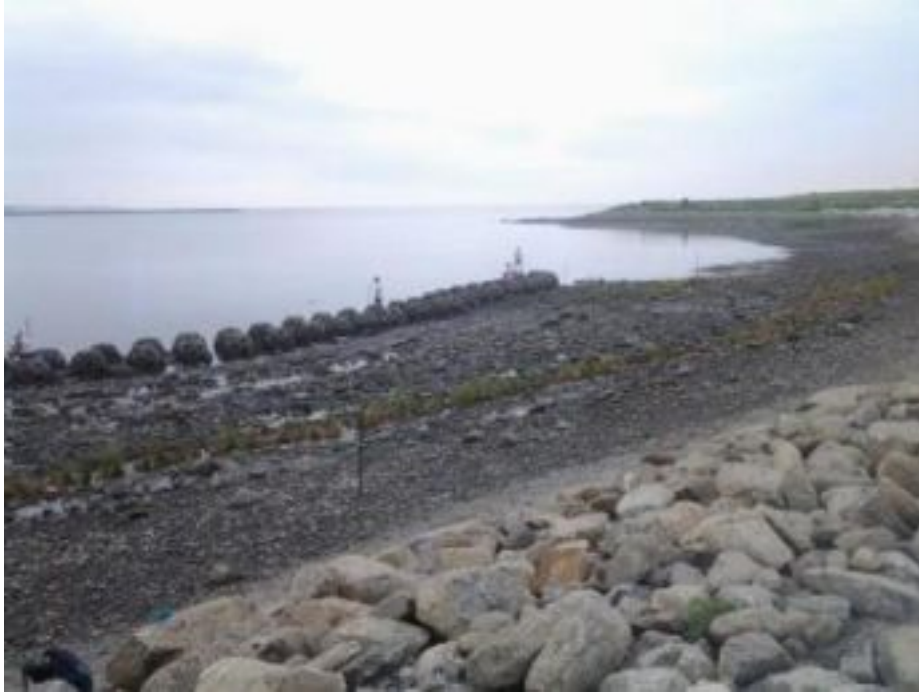
The living shoreline pilot project consisted of an artificial reef and intertidal marsh. This photograph was taken approximately three months after construction in July 2014. Note the gravel / cobble substrate.
