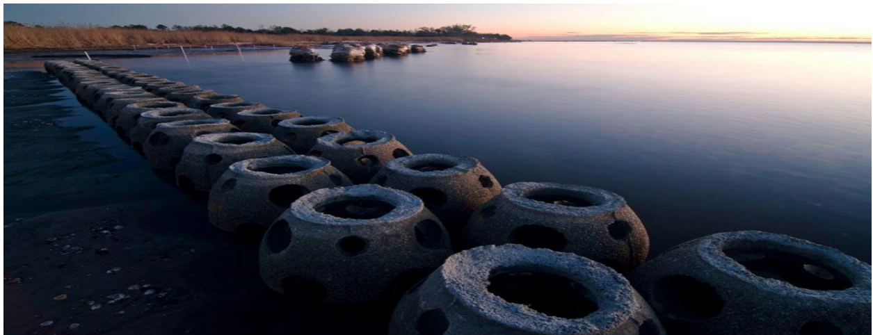
Mobile Bay Shoreline Protection with Reef Balls
