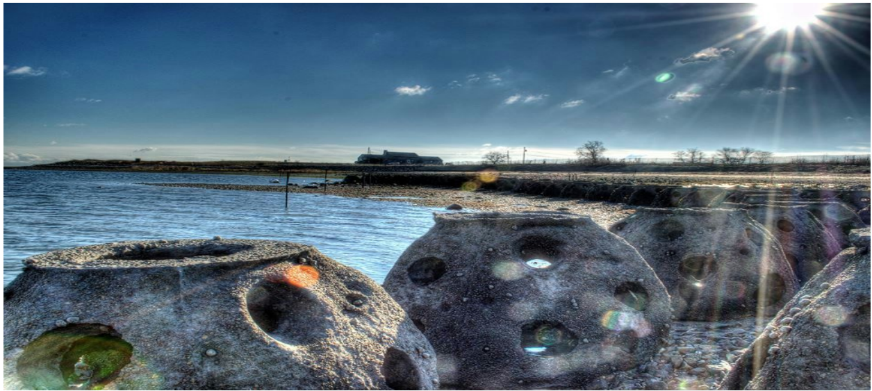
Stratford Point, Connecticut Erosion Control Project
