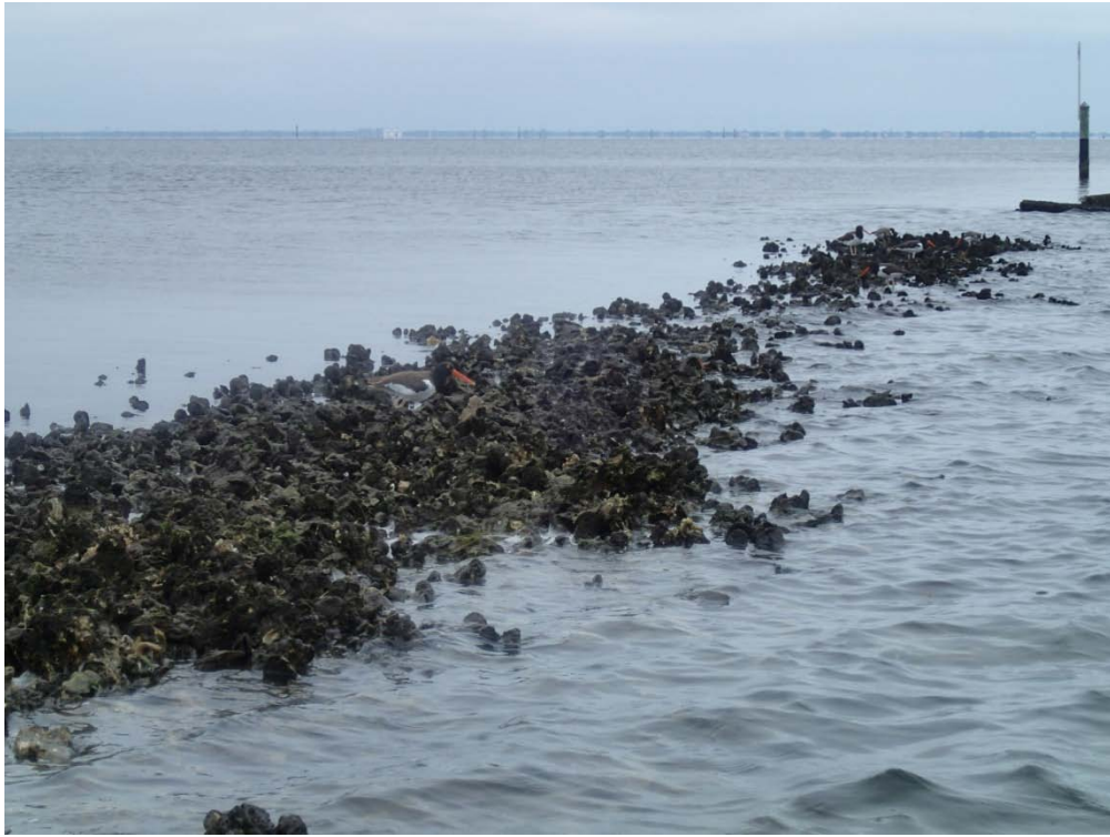
Photo 5. West end of Bar 3 (sand-filled bags covered with small riprap) facing southwest. (10/09/2013)
