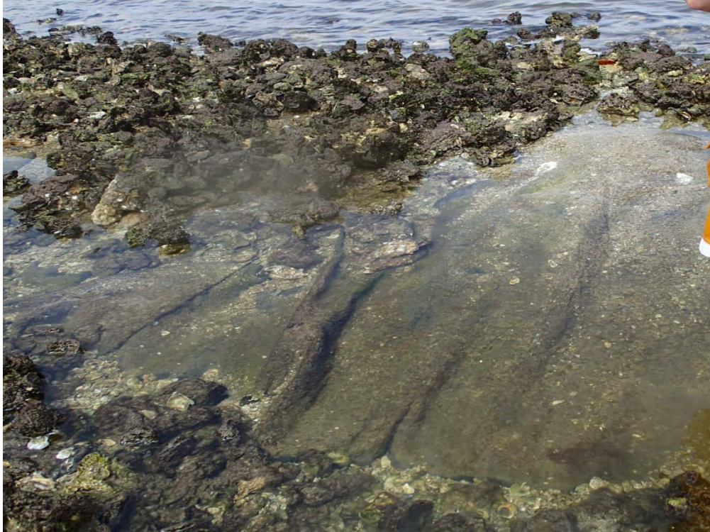
Photo 7. Bar 3 (sand-filled bags covered with small rip-rap), close up on east end of exposed geofabric (10/09/2013)
