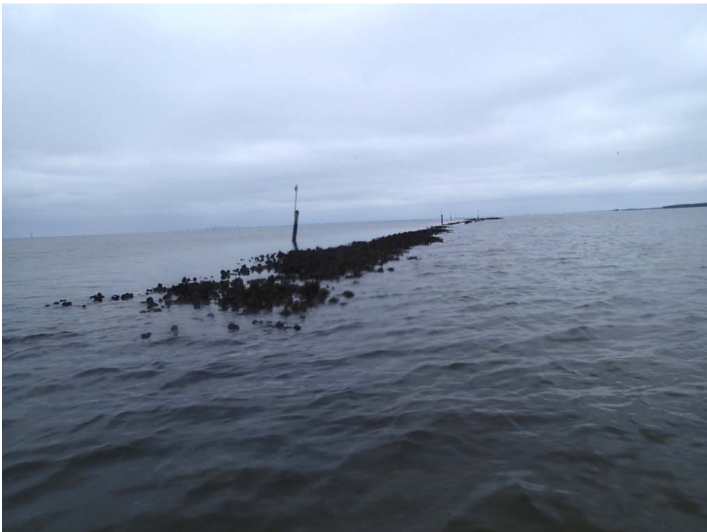
Photo 6. Representative Photo of Bar 3 (sand-filled bags covered with small riprap), facing west (10/09/2013)
