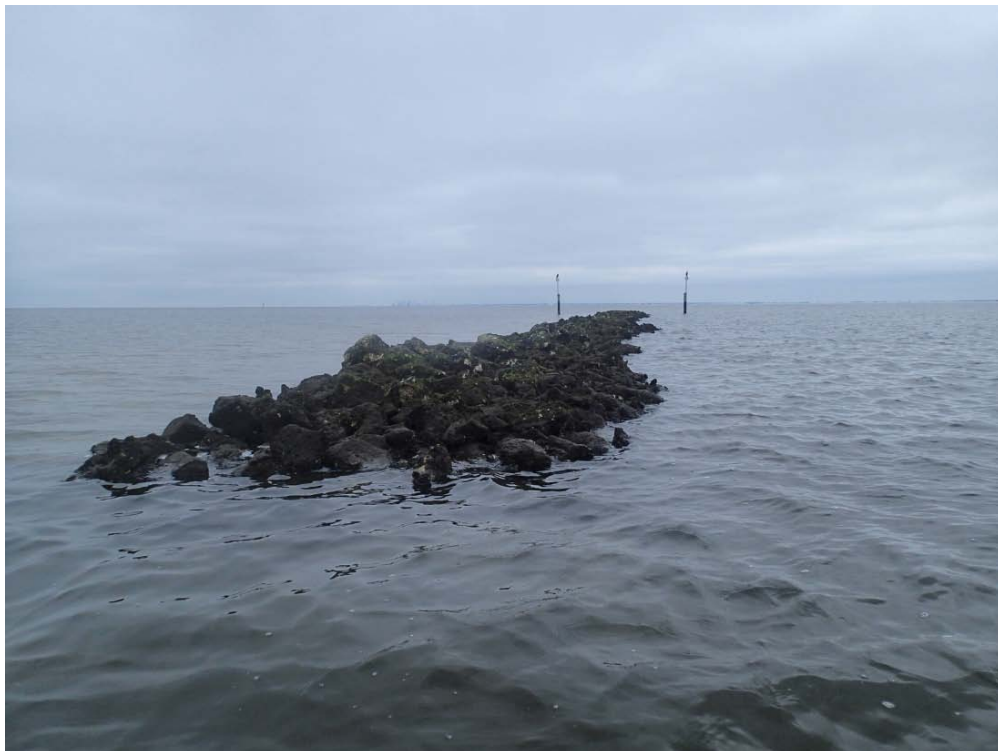
Photo 2. Longshore Bar 1 (large riprap), facing west (10/09/2013)
